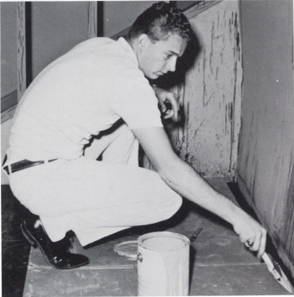
Jimmy Oates puts finishing touches on the Brewster home.
